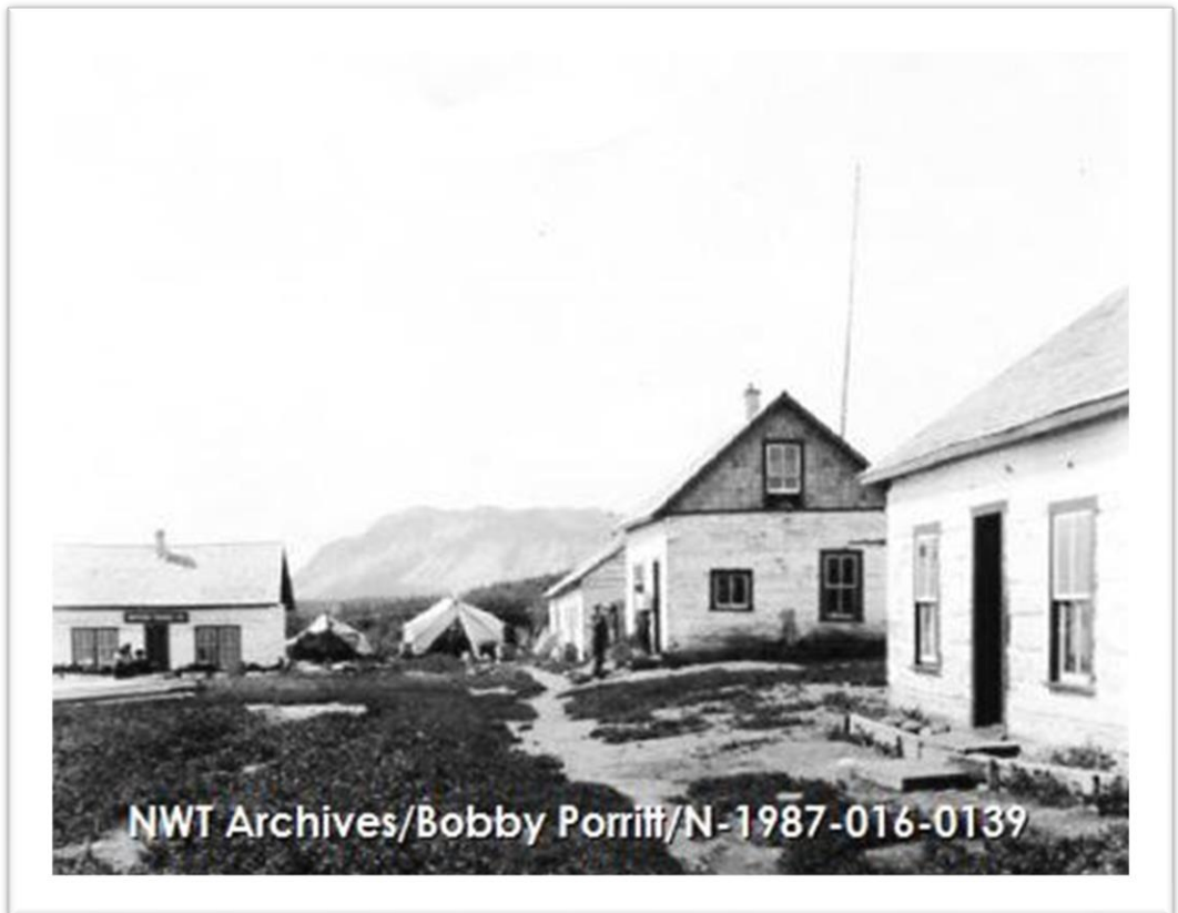
Fort Norman, 1928. Photo by Bobby Porritt.
